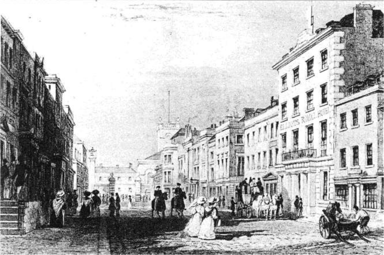
Fore Street, Devonport, in 1831 showing the entrance to the dockyard in the distance.
